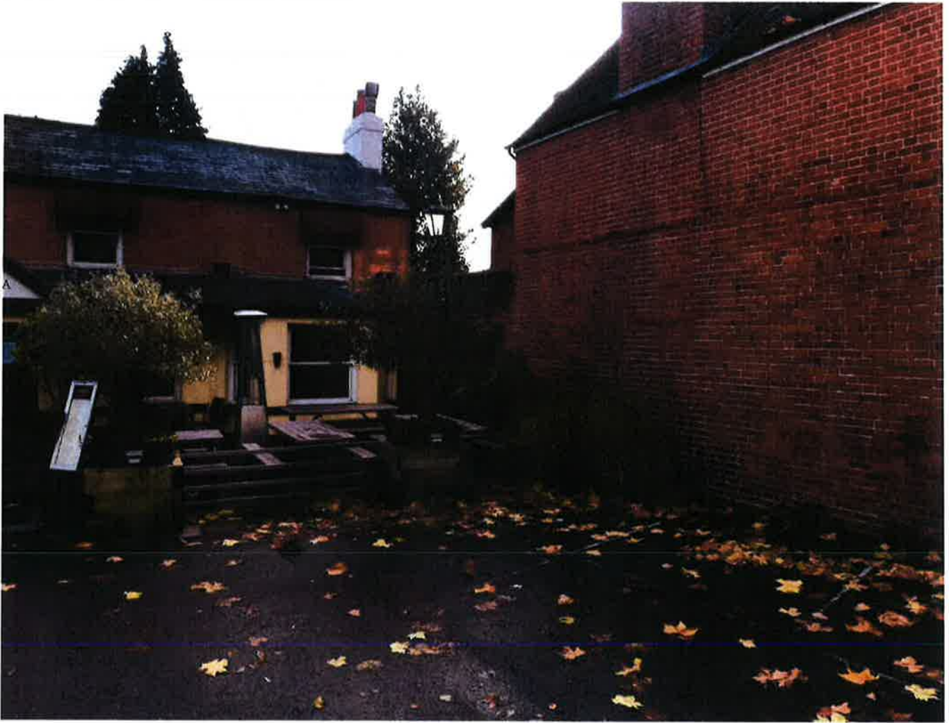
Picture 3 Side of Crossways Cottage
